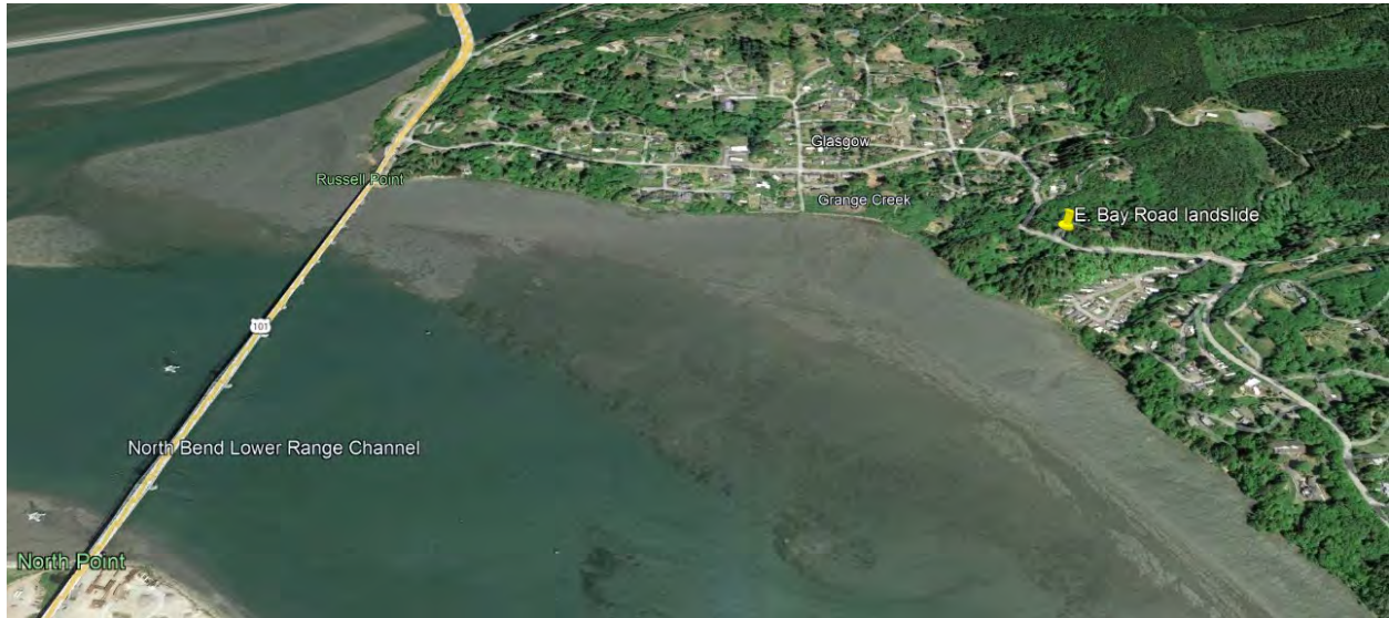
Figure I-25. E. Bay Road Landslide Location
