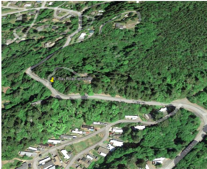
Figure I-26. E. Bay Road Landslide Intersection
