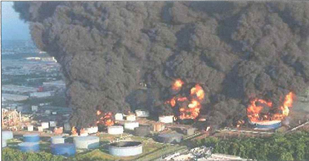
Smoke pours from petroleum storage tanks following a 2009 explosion at the Caribbean Petroleum Corp. refinery in San Juan, Puerto Rico. The blast and fire damaged 17 of the 48 tanks at the site, and flames burned for nearly 60 hours. Photo courtesy of the U.S. Chemical Safety and Hazard Investigation Board.
