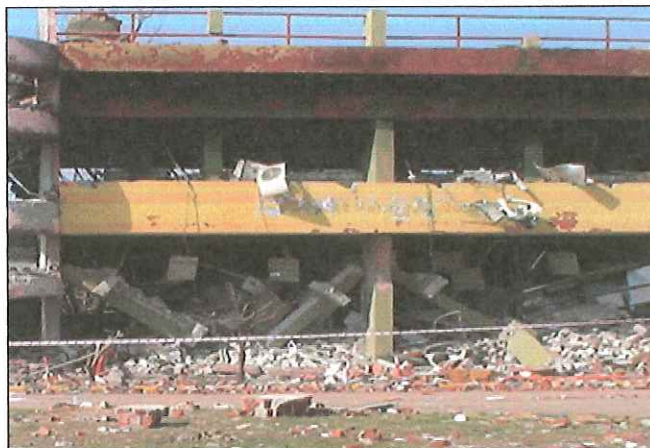
A 2009 vapor cloud explosion and ensuing fire at an Indian Oil Corp. facility in Jaipur, India, destroyed the plant and damaged homes more than a mile away, according to an investigation report. Photo courtesy of the U.K. Health and Safety Laboratory.
