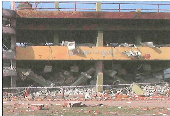
A 2009 vapor cloud explosion and ensuing fire at an Indian Oil Corp. facility in Jaipur, India, destroyed the plant and damaged homes more than a mile away, according to an investigation report. Photo courtesy of the U.K. Health and Safety Laboratory.
