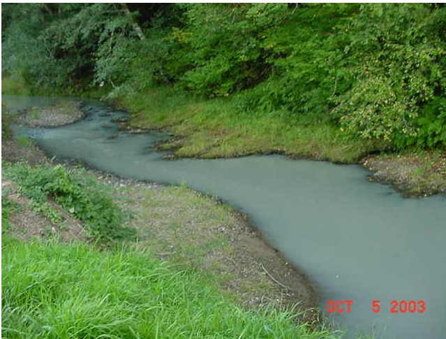
The photos above are frack-outs that occurred with the Coos County pipeline built in 2003/2004.
