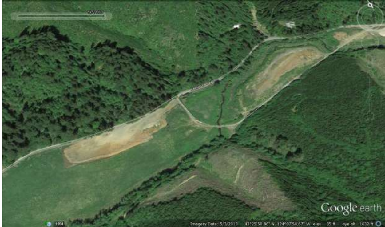
Figure 12. Fill placed between MP 3 and 4 as of May 3, 2013.
