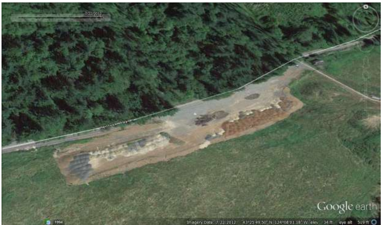
Figure 11. Fill placed south of Kentuck Way Lane between MP 3.1 and 3.3 as of July 22, 2012.
