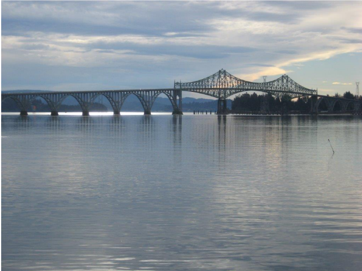
North/West side of Conde B. McCullough Memorial Bridge, North Bend, Oregon - Jan 11, 2019 - Photo Jody McCaffree
