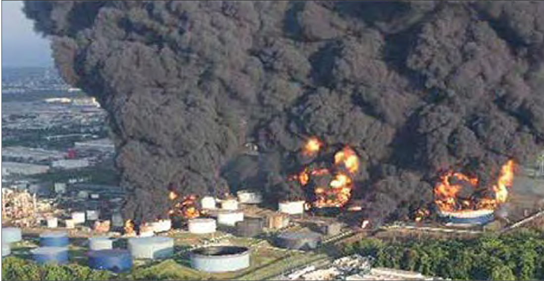
Smoke pours from petroleum storage tanks following a 2009 explosion at the Caribbean Petroleum Corp. refinery in San Juan, Puerto Rico. The blast and fire damaged 17 of the 48 tanks at the site, and flames burned for nearly 60 hours. Photo courtesy of the U.S. Chemical Safety and Hazard Investigation Board.
