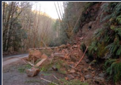
Landslide along the Smith River in the Oregon coast range.
