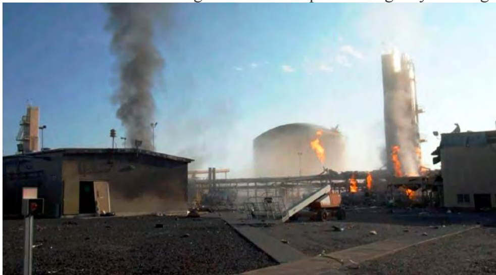
Fires burn at site of Plymouth LNG explosion. by Washington Utilities and Transportation Commission (Used with permission.)
