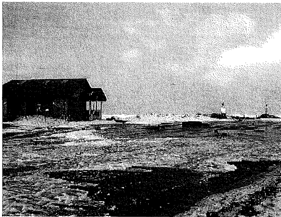
Figure 3 - December 22, 2000 Wave Runup at Bandon Wave overtopping during a major storm (22 December, 2000) surrounds the restroom and covers the parking lot adjacent to the south Coquille jetty at Bandon (Photos courtesy of Dr. J. Marra, pers. comm., May 2010).
