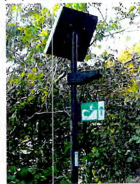
Figure 4. Use of solar panels help to illuminate signs during night time.
