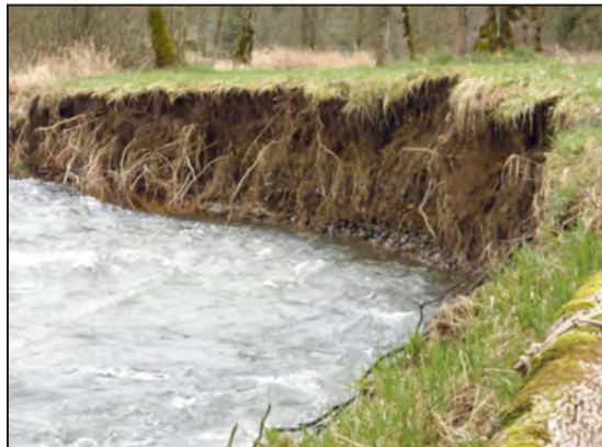
Figure 29. An eroding stream bank on the Oregon coast, which has been facilitated by the removal of stream bank vegetation. Source: Clackamas County Soil and Water Conservation District 2015
