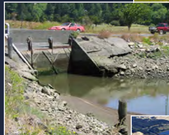
Kentuck Slough levee and tide gate
