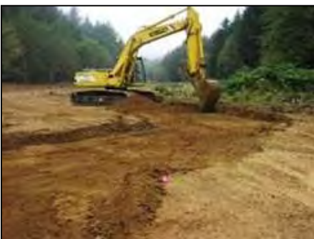
Figure 13. Excavation of the Anderson Creek high flow channel in the regraded Anderson Creek floodplain.
