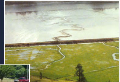
Haynes Inlet levee
